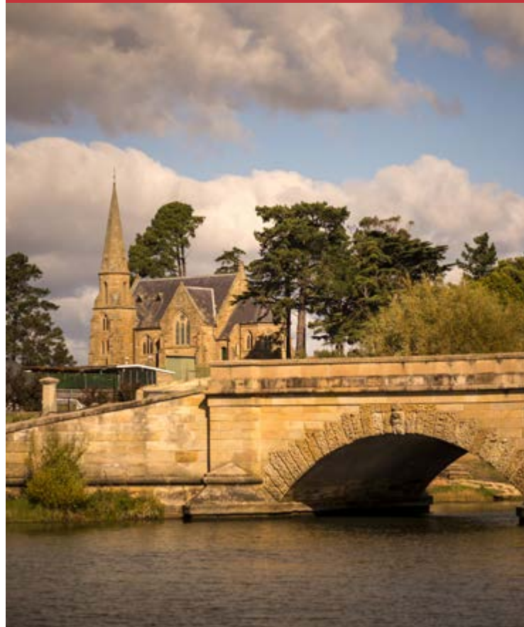
The bridge at Ross (credit Tourism Tasmania & Rob Burnett)
